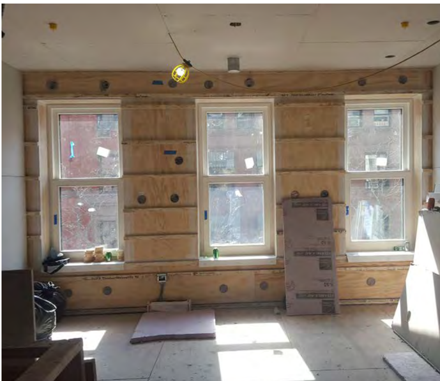
PROCESS OF EXTERIOR WALL INSTALLATION / AIR BARRIER APPLICATION
