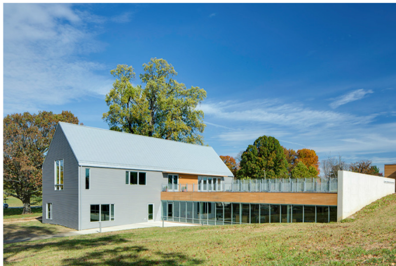
Headquarters building (10,000 SF)
