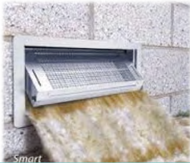
WET FLOOD PROOFING - Passive
