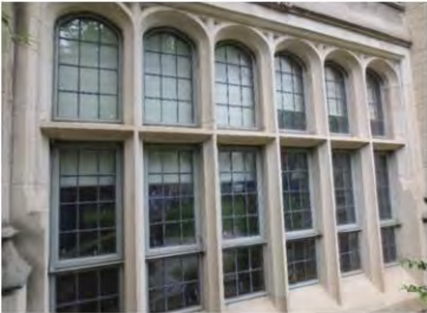
IMAGE 11: TYPICAL RESTORED PODIUM WINDOWS (EXTERIOR VIEW)
