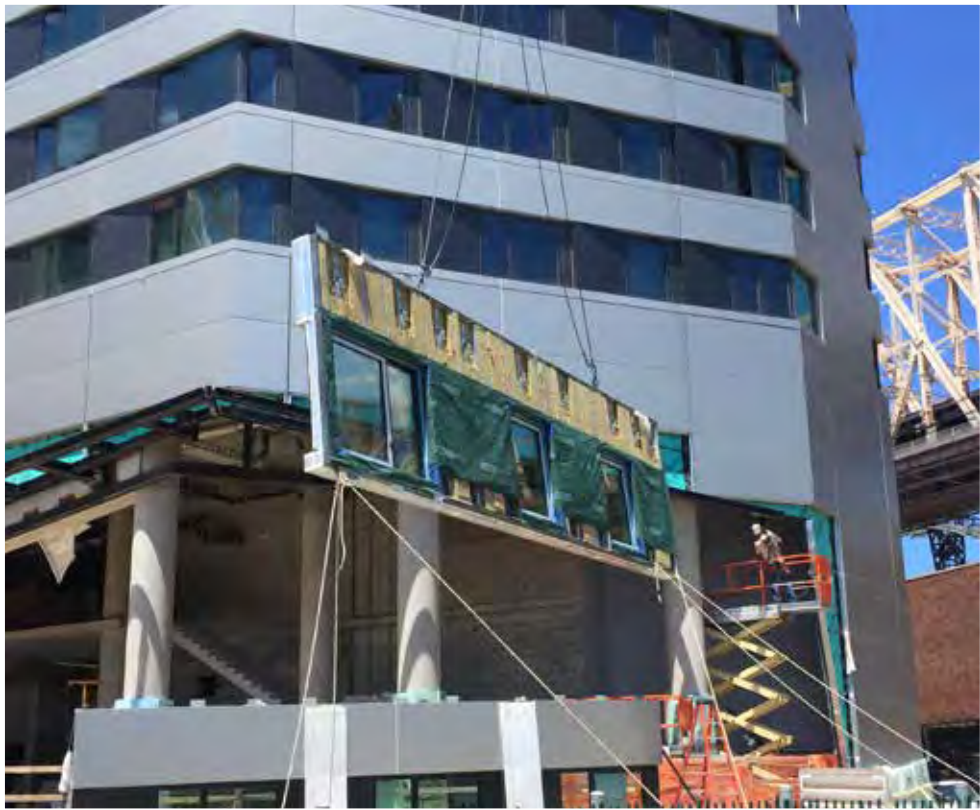
Prefabricated metal wall panel installation
