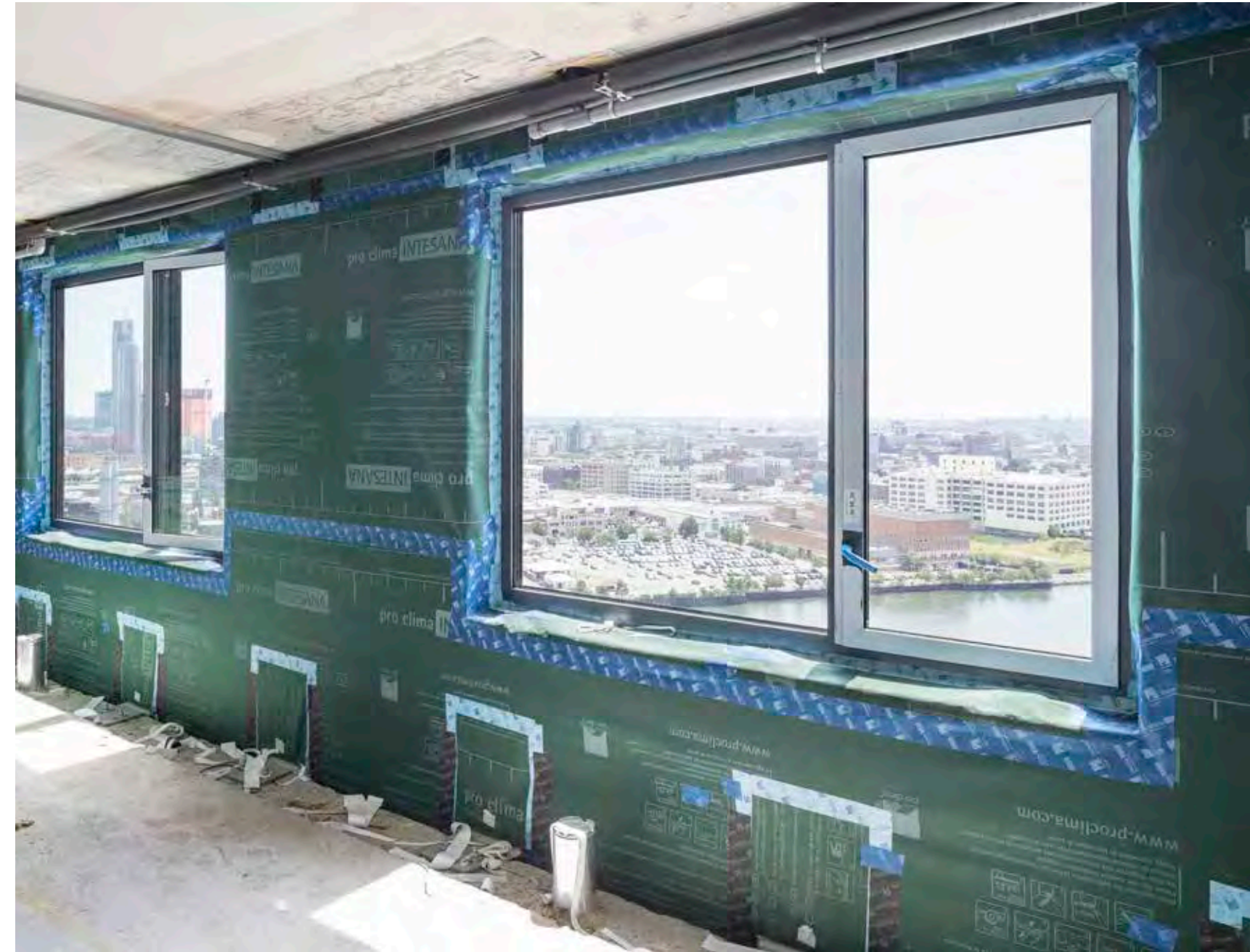
AFTER PANEL SUPPORTS SEALED
