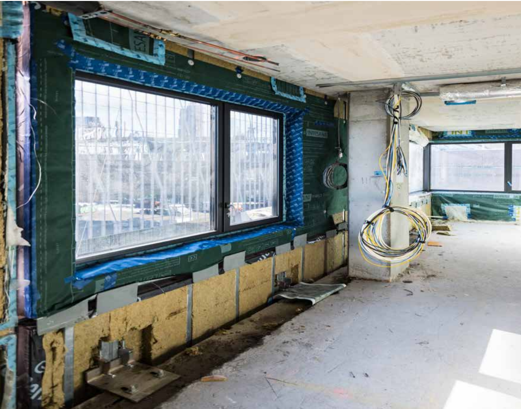
BEFORE PANEL SUPPORTS SEALED
