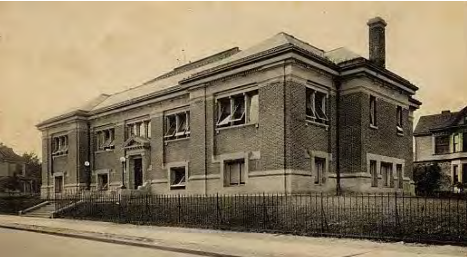
East Branch Library c. 1914
