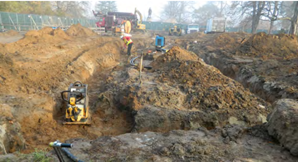
Geothermal Field Installation
