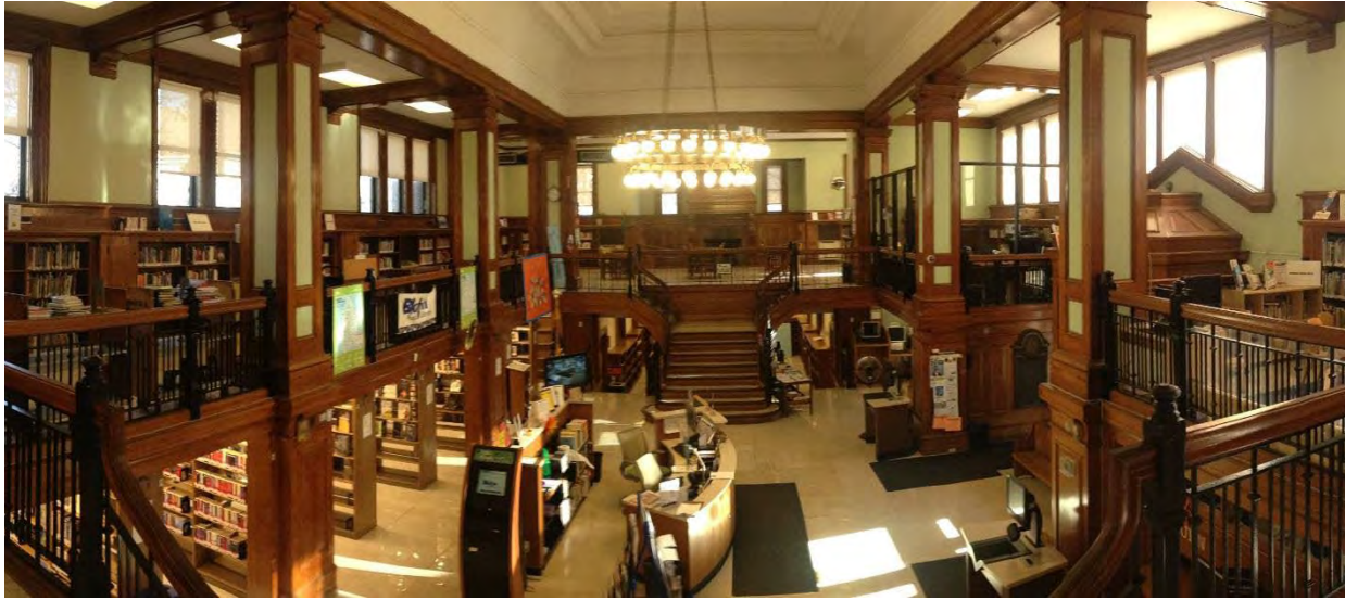
Built-In Bookshelves Preclude Wall Insulation
