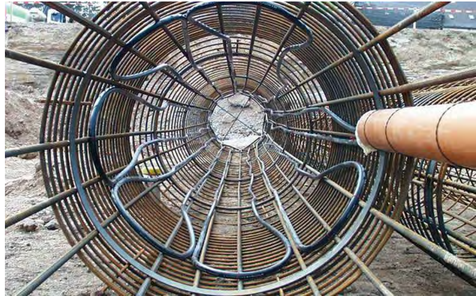
Geothermal Pile Frame
