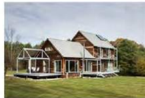
FARMSTEAD PASSIVE HOUSE Certified Passive House | 4.5kBtu/sf/yr
