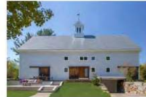
RYE BARN RENOVATION Barn Residence Deep Energy Retrofit
