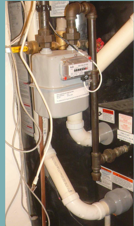
Small natural gas meter on Versa Hydro for breaking out gas from solar thermos
