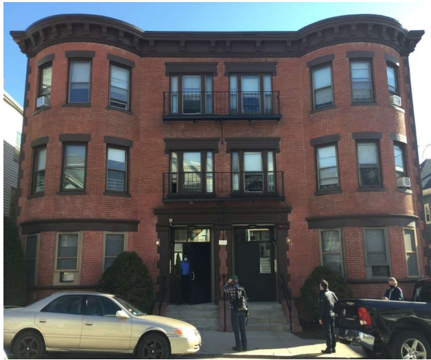
Type 2 - Small Masonry building with square footage below 25,000 sf.
