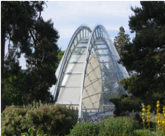
THE ALPINE HOUSE AT KEW WILKINSON EYRE C 2006
