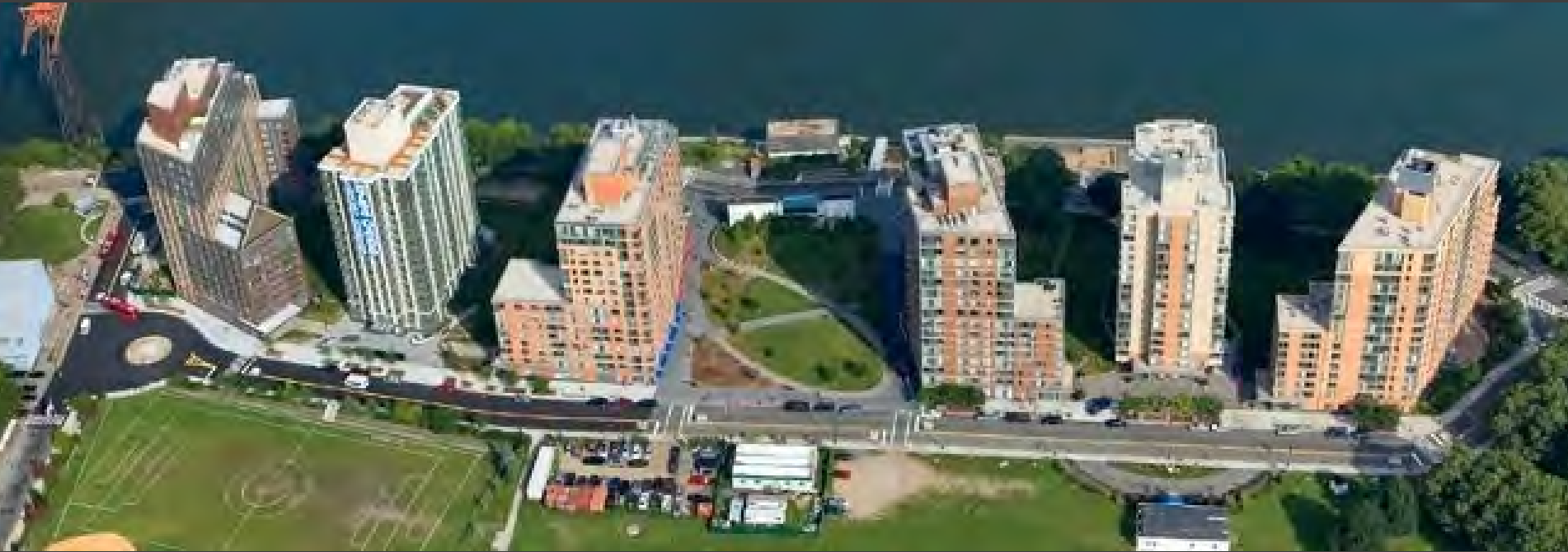
Seven Buildings on Roosevelt Island
