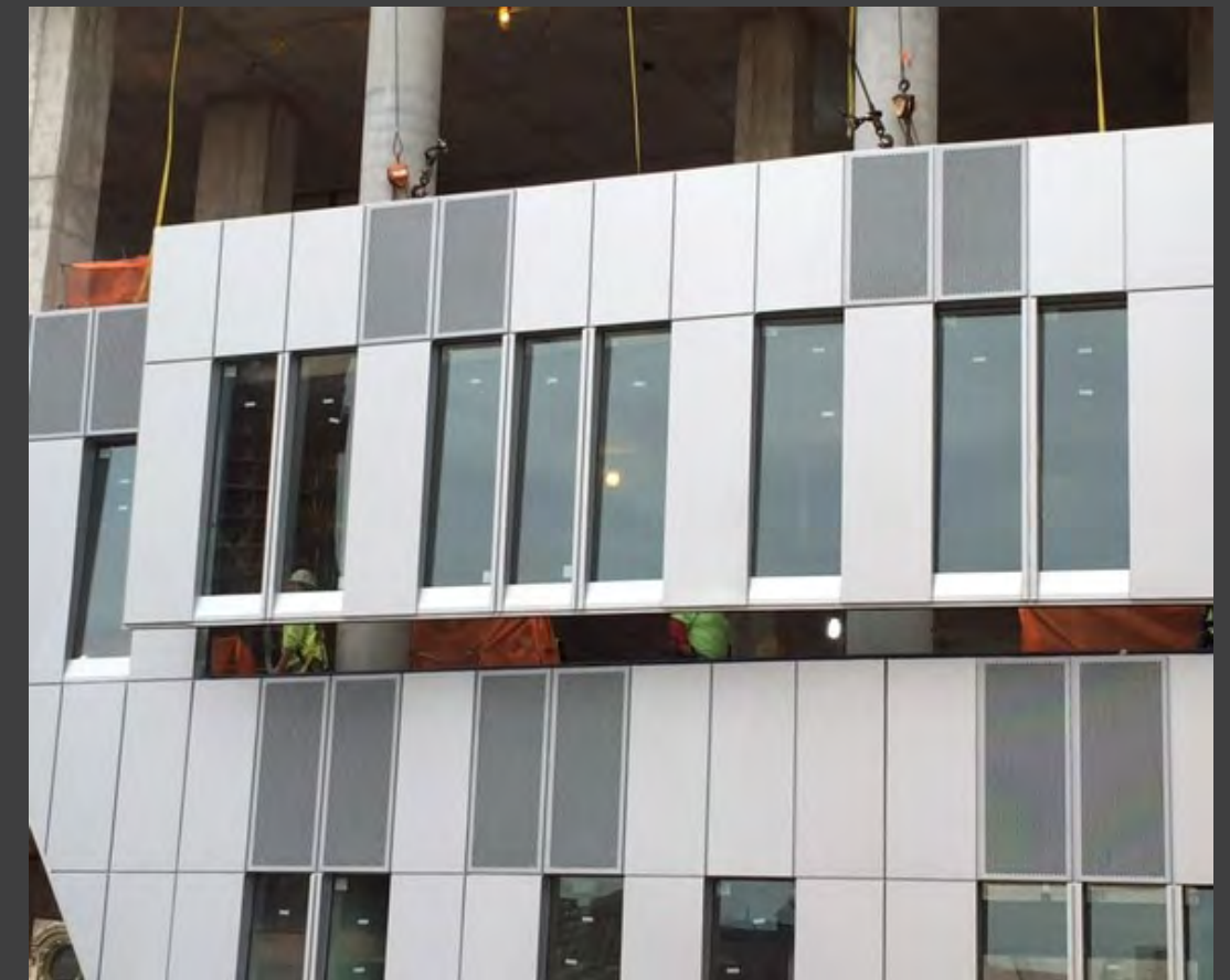
Prefabricated metal wall panel installation
