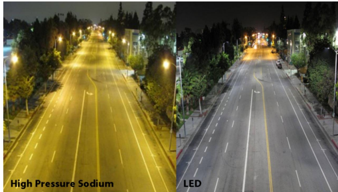
High Pressure Sodium Los Angeles' Hoover Street before ... Credit: Los Angeles Bureau of Street Lighting
