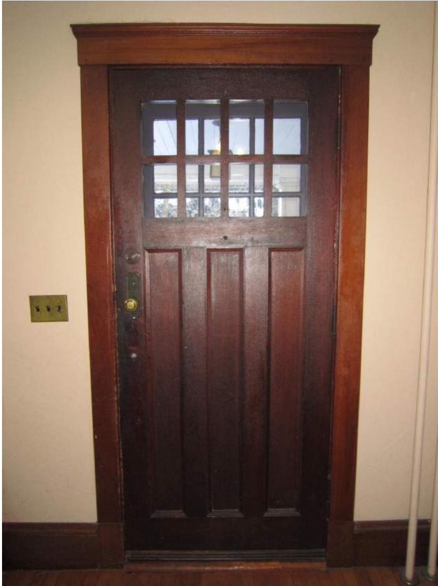
Thermal bridging at the front door- FROST-new storm needed
