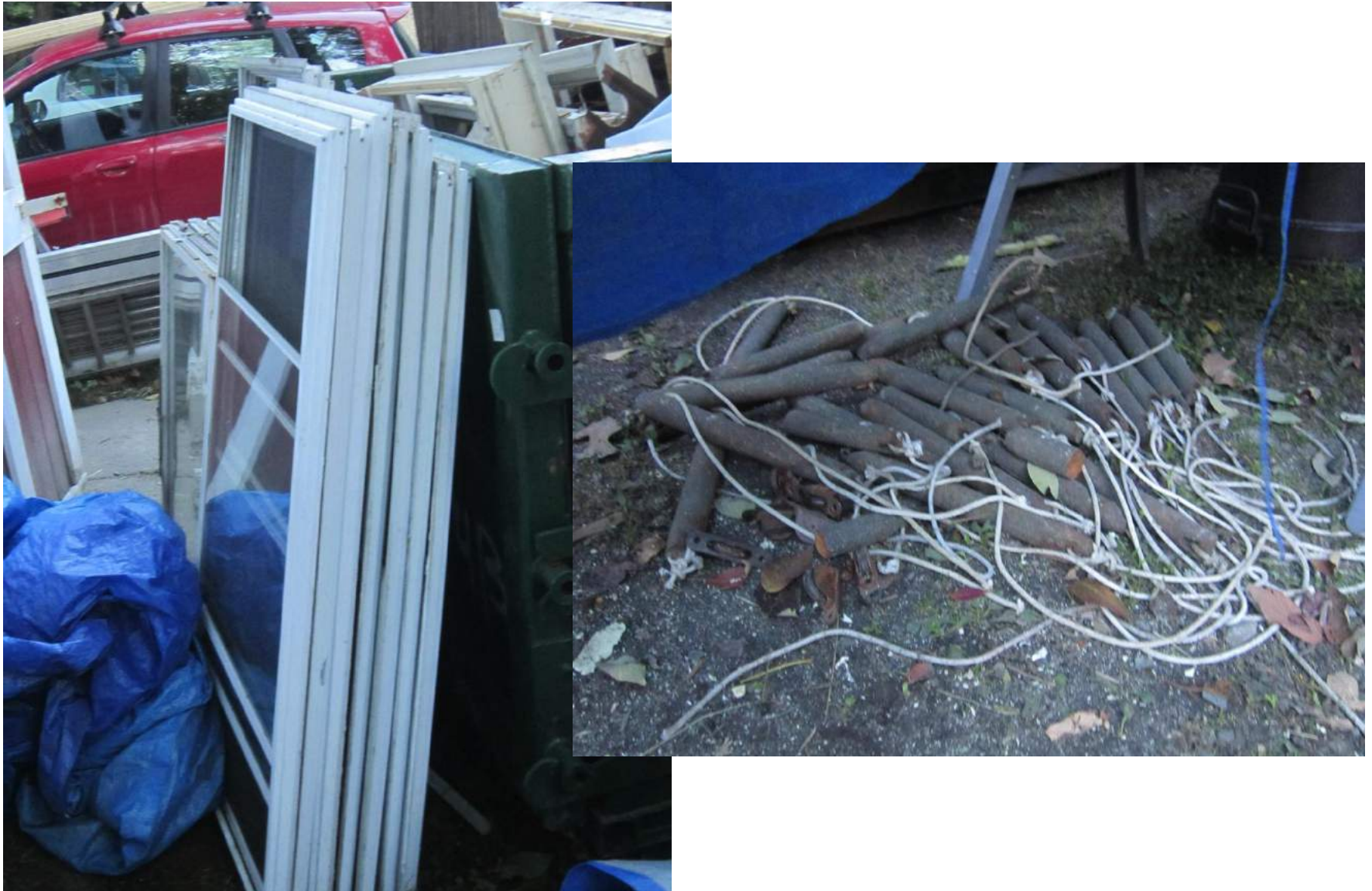
Storm windows salvaged for re-use and window weights to scrap metal
