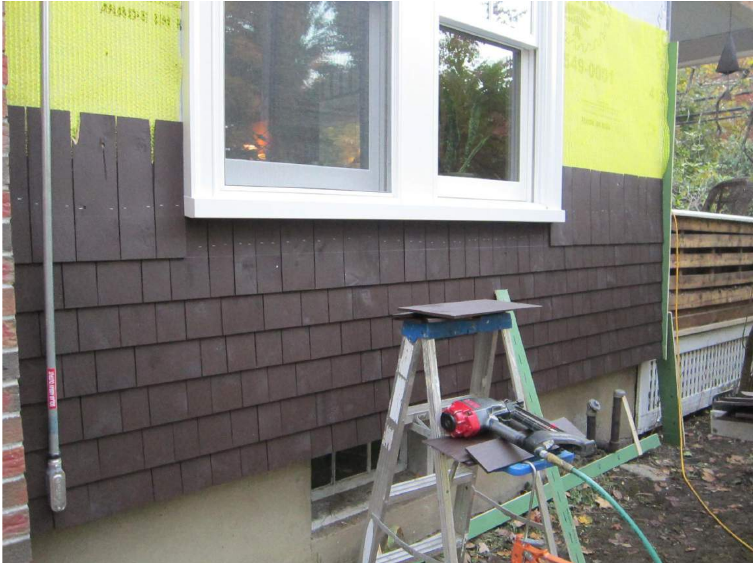
Pre-stained shingles to match original going on
