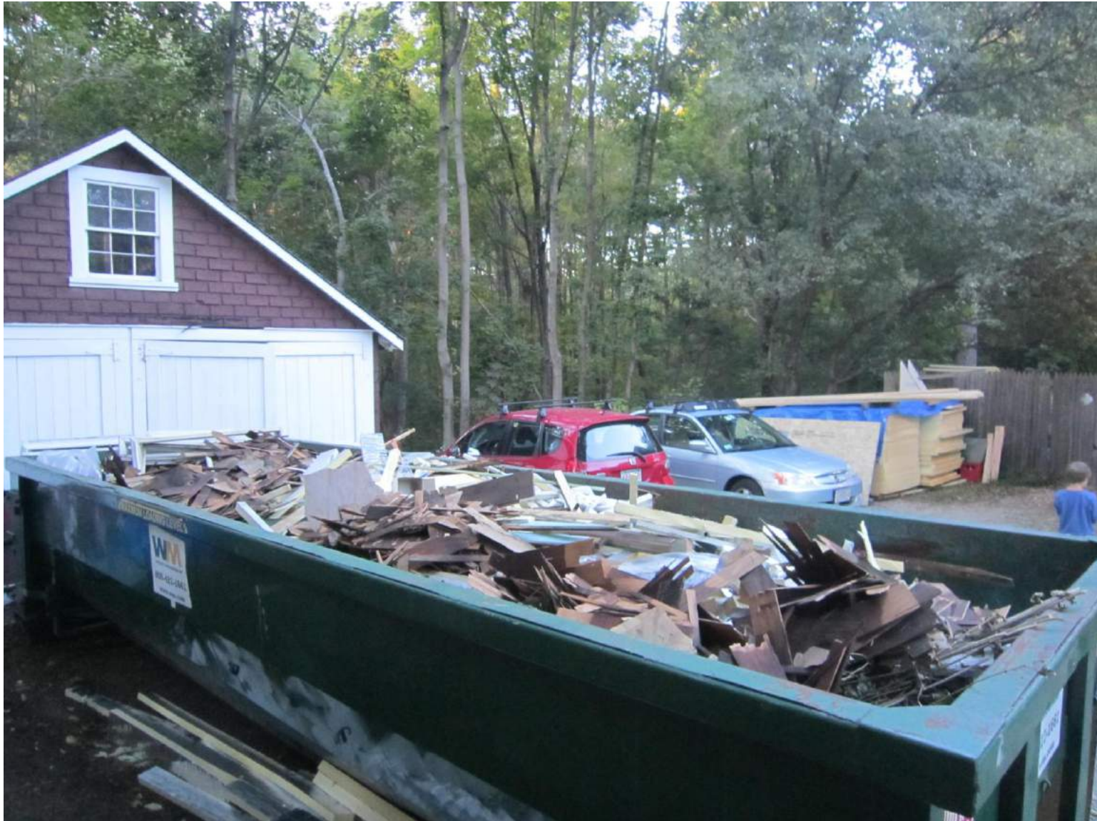
Old shingles go to the dump- salvaged from bathroom for garage
