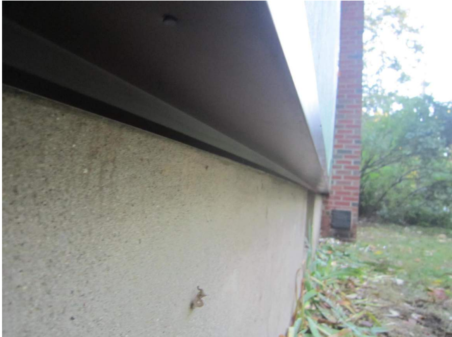
Break metal flashing sealed to foundation wall to protect foam
