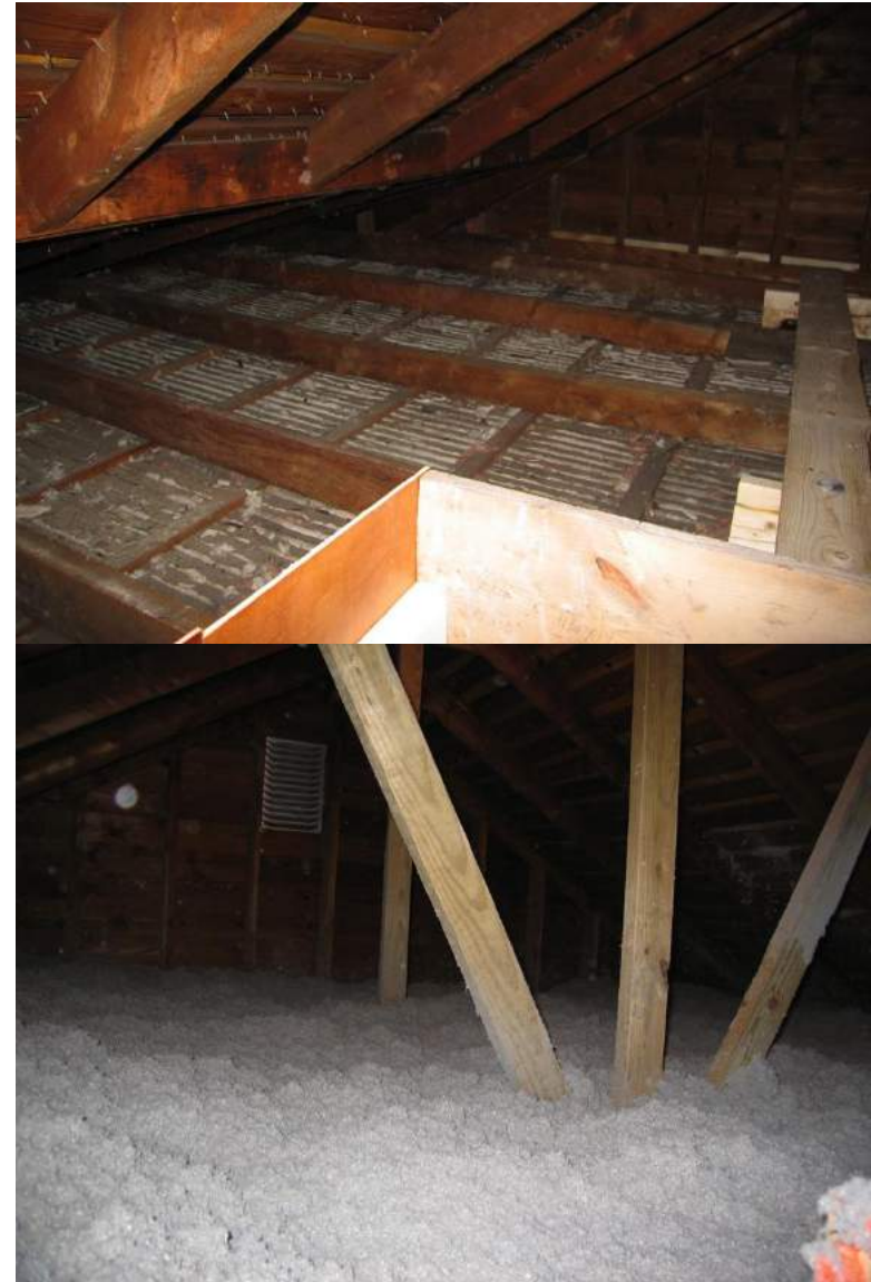
2008- Remove all the old insulation (tiny hatch) and Insulate the attic
