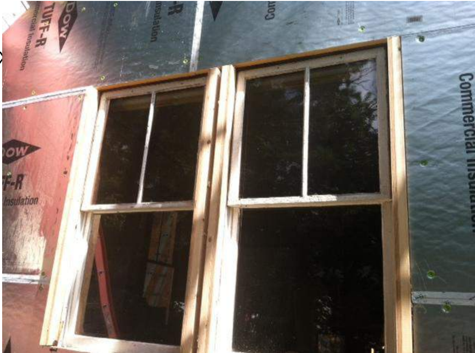
Minimal disruption- sashes stay in place until new unit installed
