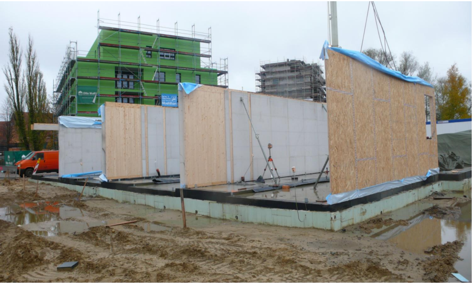
pre-fabricated solid wood panels on site
