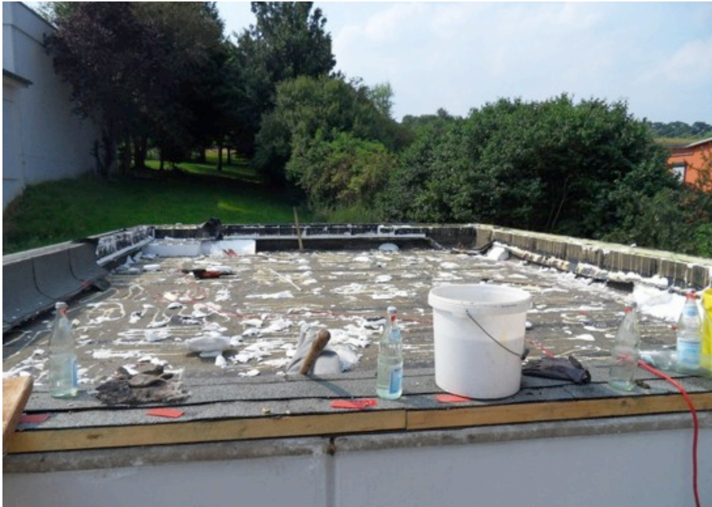
demolition work - roof
