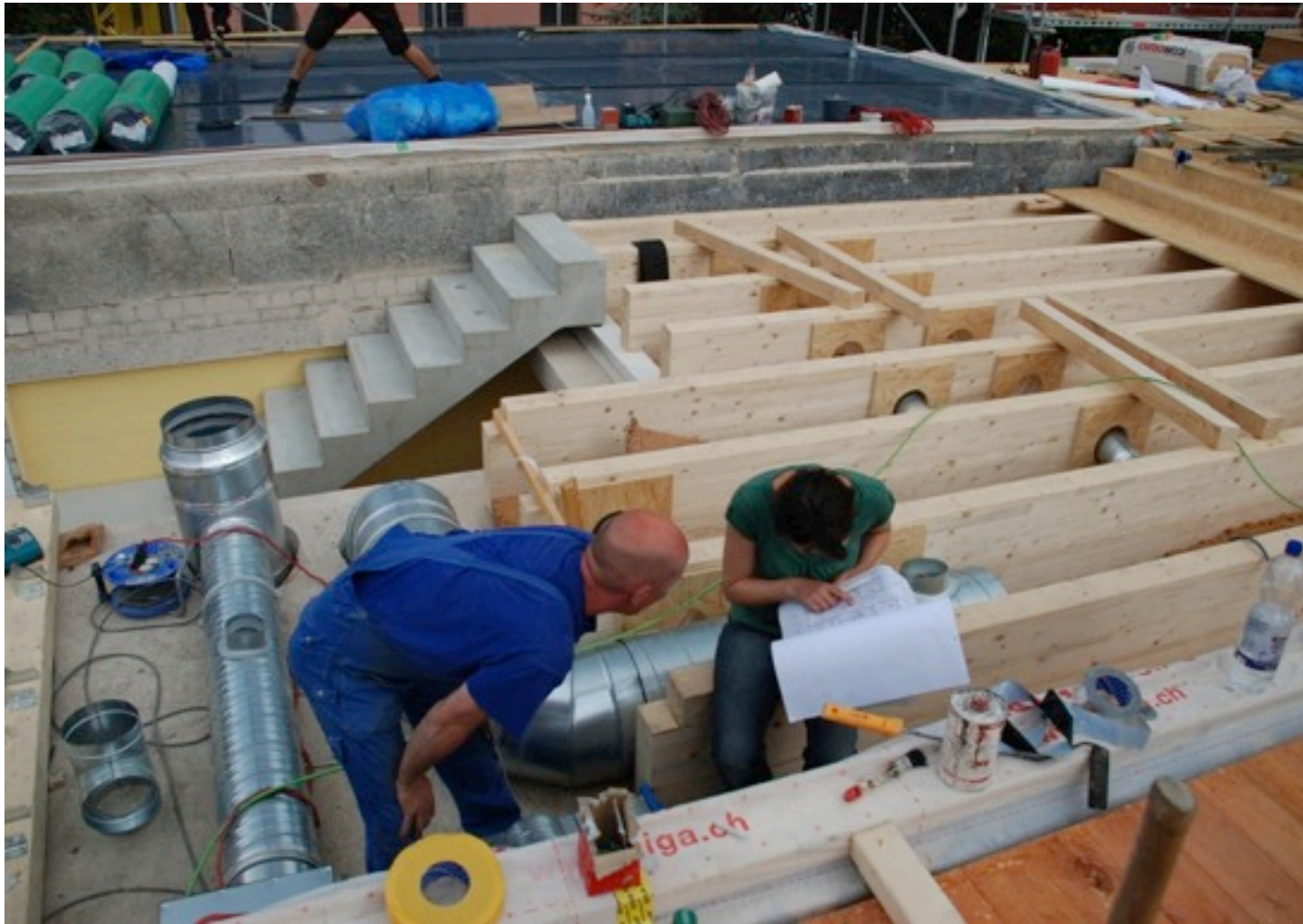
joint connection: ventilation on top of the entrance
