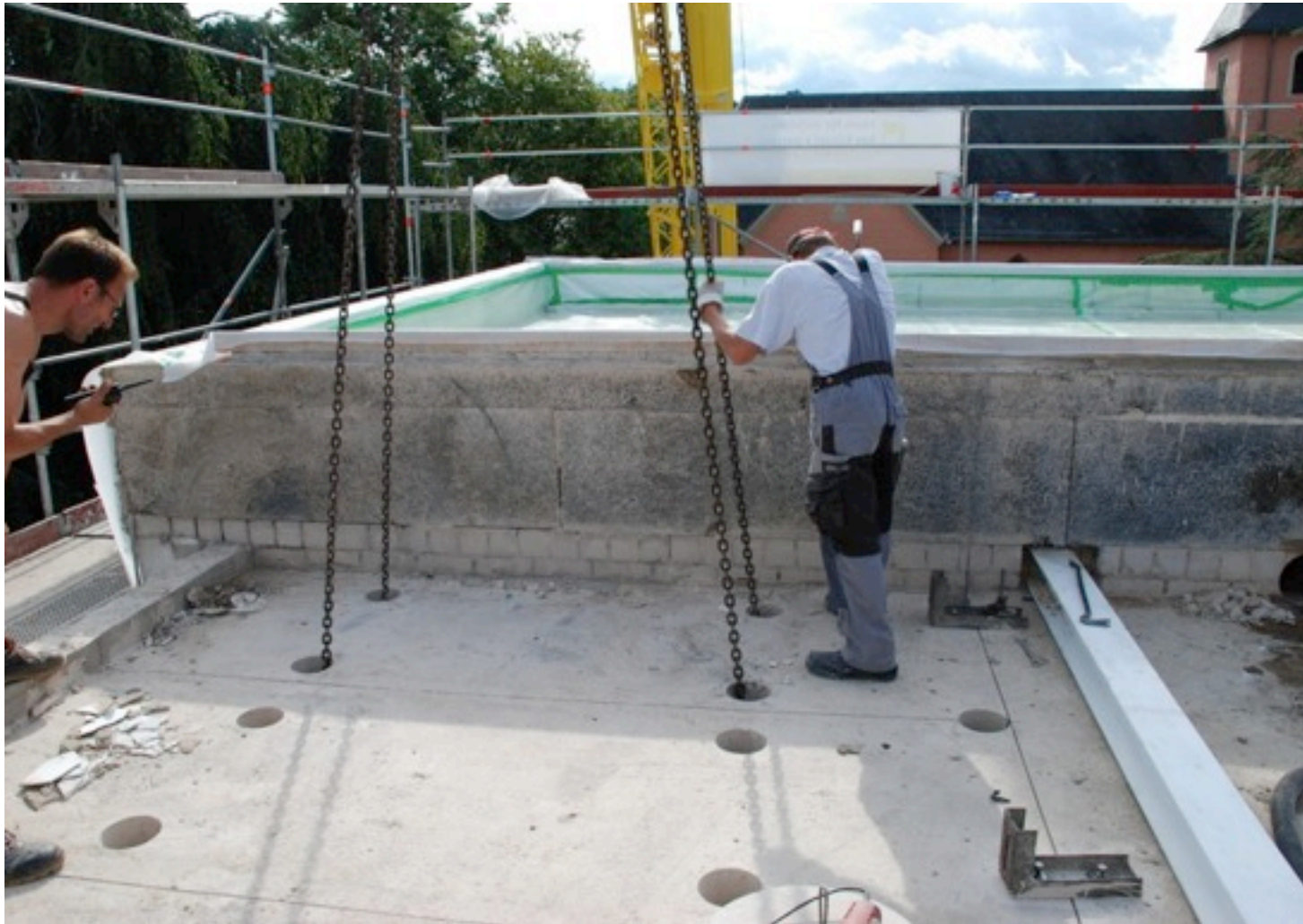
breakthroughs for staircase
