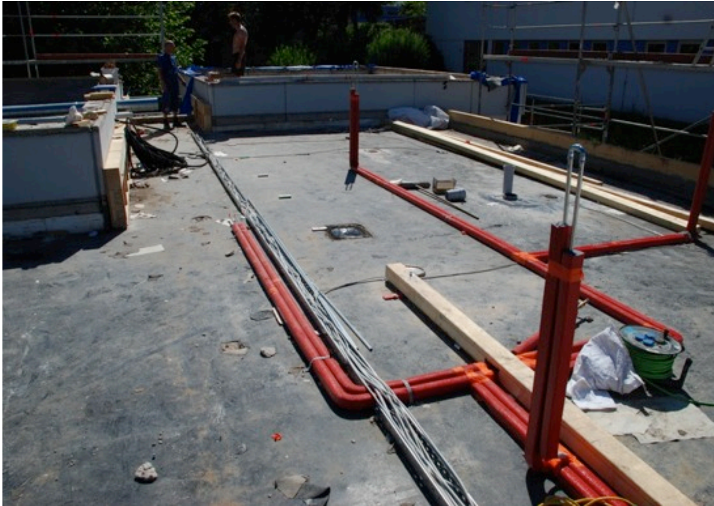
cable running according to detailed planning
