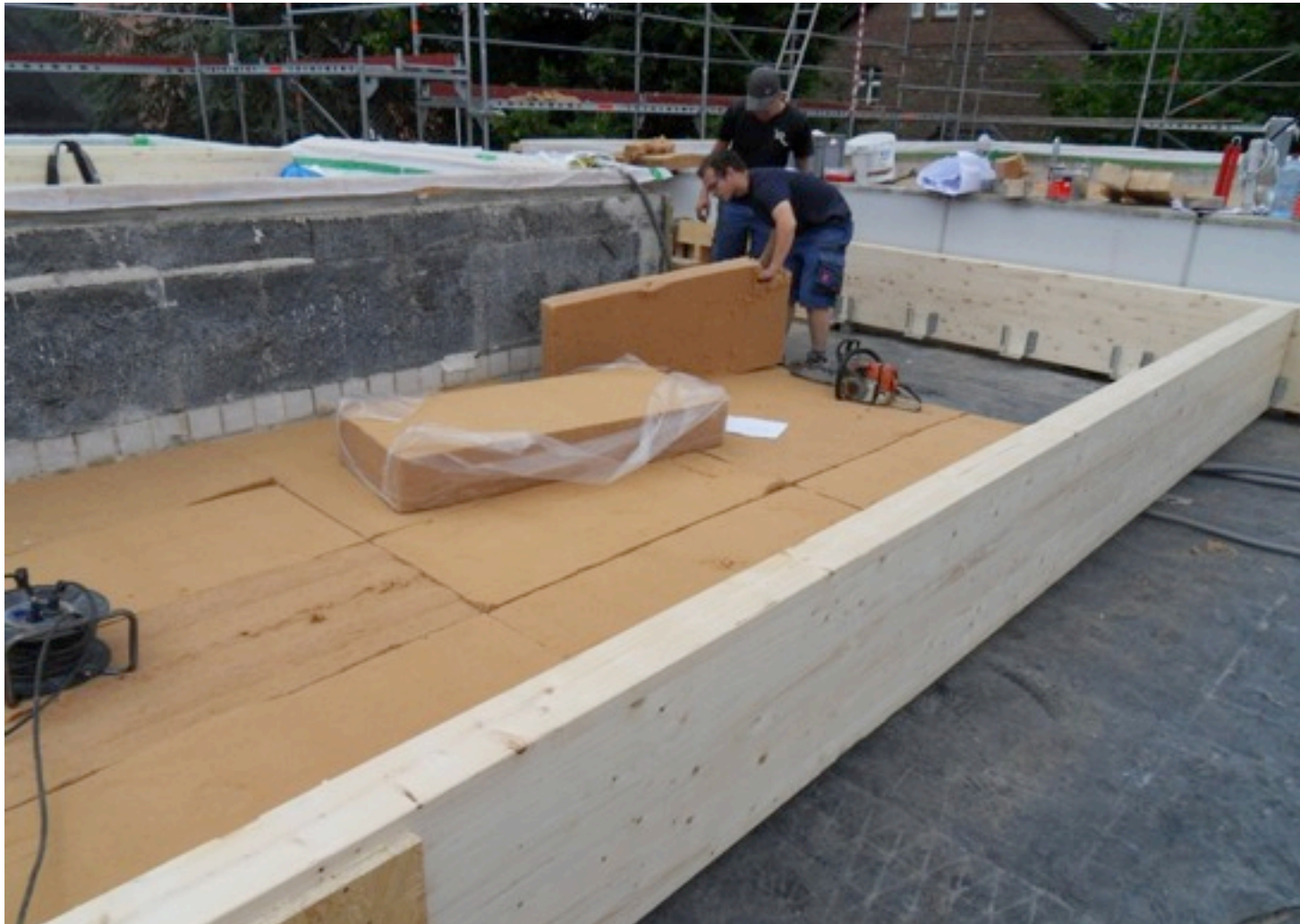
frame of joists
