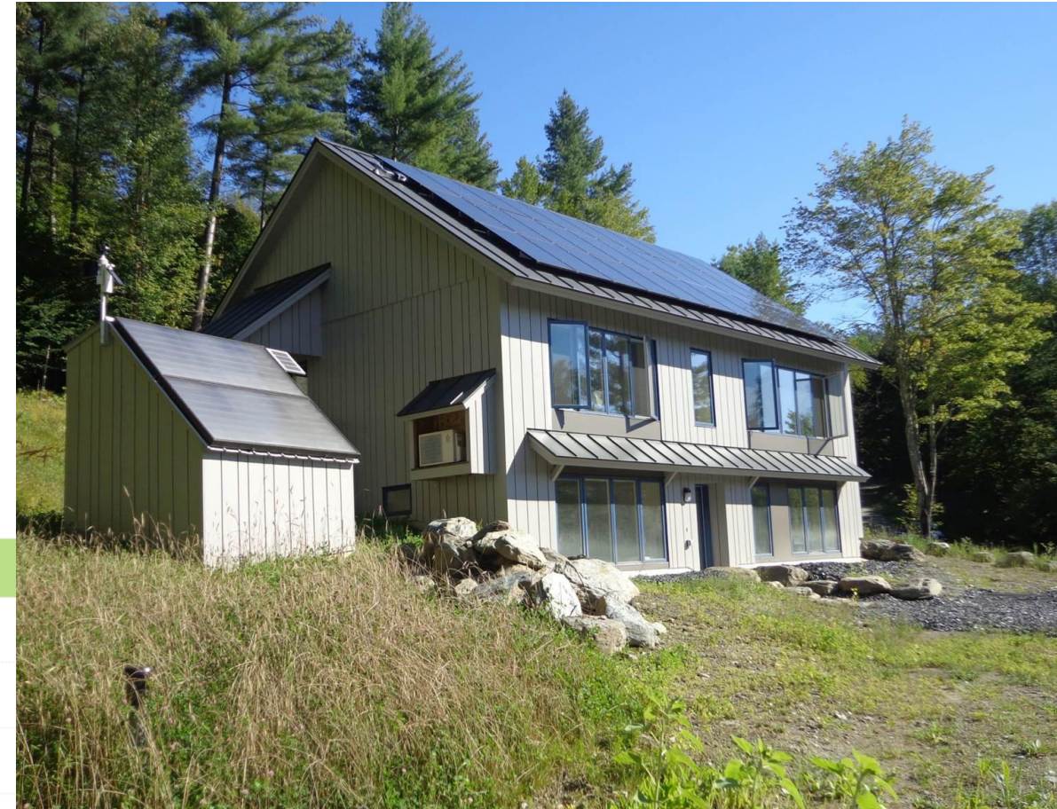
Photo courtesy of Turtle Creek Builders, Waitsfield, VT
