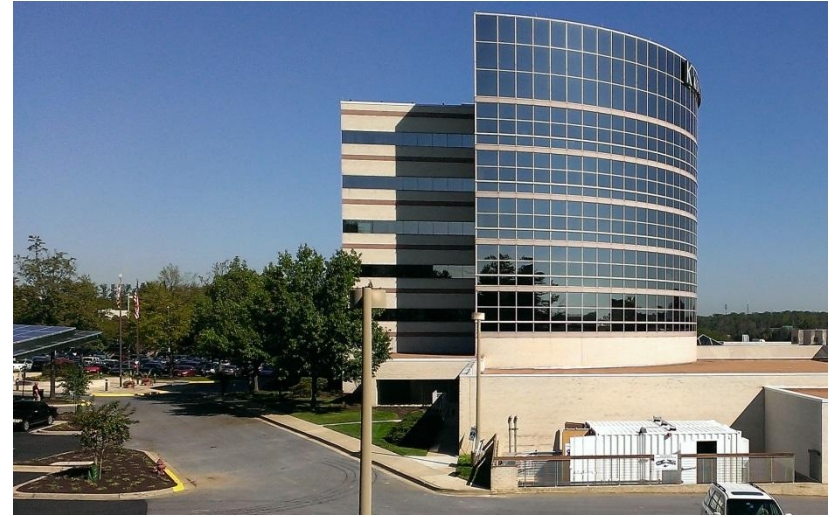
Konterra Headquarters Laurel, MD – 500kW
