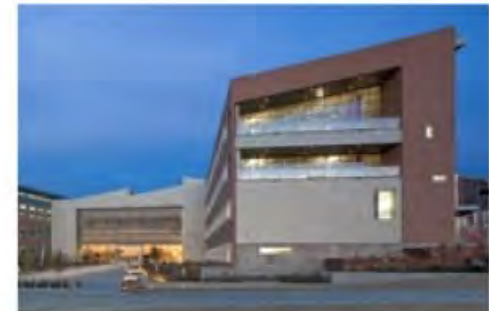
Large Office Facilities
